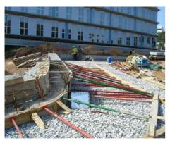
The east path is built on the roof of an existing underground parking. This path rests on a green topography with a slight slope towards south. This new acces is designed as a carpet made of prefabricated concrete pieces placed on the compacted ground. A continuous bench made of reinforced concrete accompanies the green slope that hides and integrates the element of ventilation of the underground parking.
