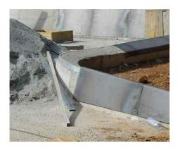
The path from south is defined by some irregular reinforced concrete walls that relate the existing conditions and topography through its organic gestures. The walls, covered with a corten steel plate siding, allow the pass of the flagstone path through the green areas, as if it was a dug furrow. The corten steel plates fold itself to generate linear benches in the small areas of square.
