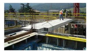
The building structure is made with reinforced concrete. The horizontal structure is solved with prefabricated lightweight slabs. These slabs, with a span of 12 meters, are able to solve the multipurpose hall without intermediate columns. This structure is trimmed by its interior edge in order to allow natural crossed ventilation and the entrance of natural light to the rear part of the hall.
