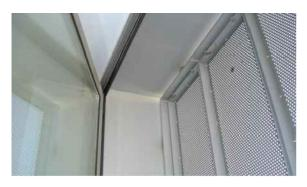
Just like architecture is studied to improve the use of natural light, different constructive solutions are applied to introduce solar control: at south fibreglass roller blinds and at east and west drilled steel plate shutters.
