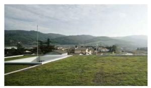
The green roof is treated as part of the landscape and includes a "gramma" plantation, with a low water consumption, that grows on 10 cm of rich soil. The rest of the flat roofs are a floating ventilated floor where several horizontal skylights introduce natural light to its interior to reduce the electric consumption on artifical lighting.
