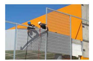
A new metallic structure is superimposed to the existing concrete roof to achieve a more regular shape. The perimeter of the lower slab is completed in order to define exterior courtyards that include green areas with trees. The process of construction it is alternated with the deconstruction one to adapt to the pre-existing conditions. In the first phase the scattered existing services on the roof are repositioned in a new space with the new ones.
