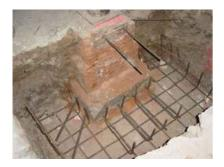
Foundations and floor slabs are reinforced in order to assume new loads. Unidirectional floor slabs are reinforced with a new compression layer of concrete connected to beams through metallic connectors. Thermal insulation is applied to façades through an interior plasterboard cladding. The new aluminium windows include self-regulated airflow systems to
