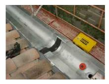
The roof is renovated with recycled tiles and new ventilated ones in order to generate a new ventilated chamber and thus the thermal conditions improve and the air-conditioned volume is reduced. New zinc rainwater-pipes and guttering are added. The new south gallery is built with dry construction systems and the building services are designed to integrate in the pre-existing architecture.
